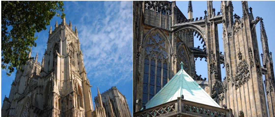
Fig. 1 Exterior of the buildings.
